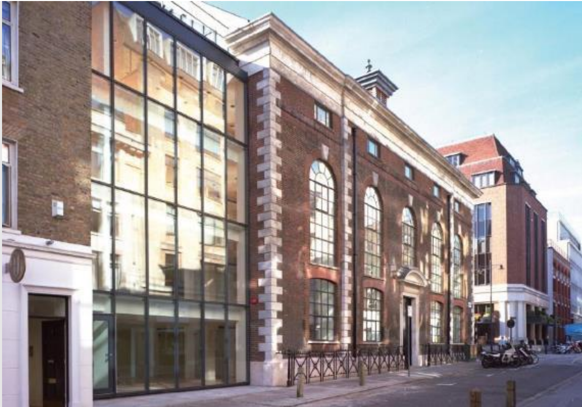
Figure 98 - Wren House, Hatton Garden: Originally built as a church in c.1670, it was then adapted for use as a charity school in 1696, before being reconstructed internally to provide contemporary office space. The original Grade II listed facade has been restored and retained.
