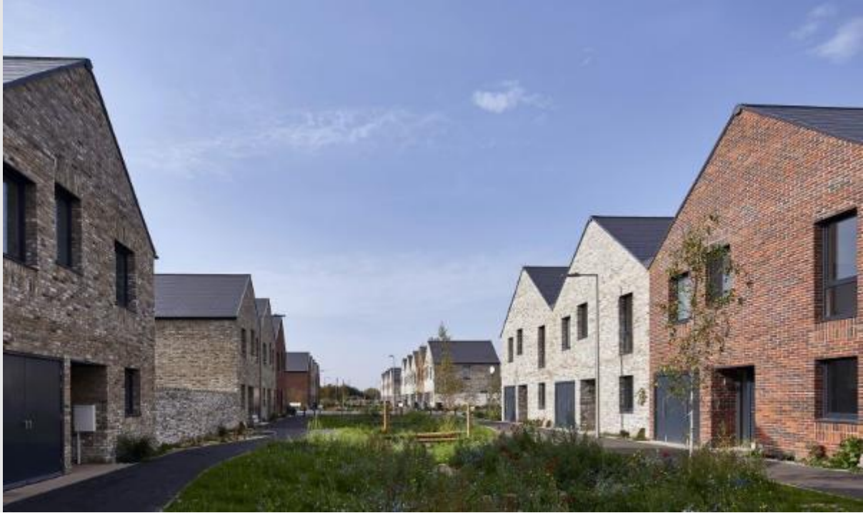
Figure 26 - St Chad's, Tilbury: Traditional pitched roof forms with high quality materials and detailing create a familiar but contemporary feel.
