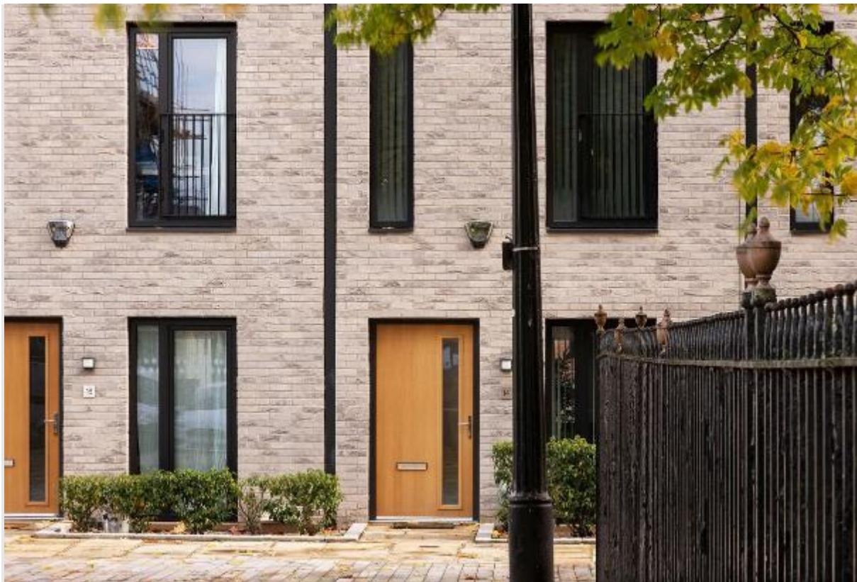
Figure 29 - Timekeepers Square, Salford: A limited materials palette is used throughout the scheme; predominantly a light brick in response to the sandstone of the nearby Grade II listed church. The materiality and architectural detailing is simple and restrained.
