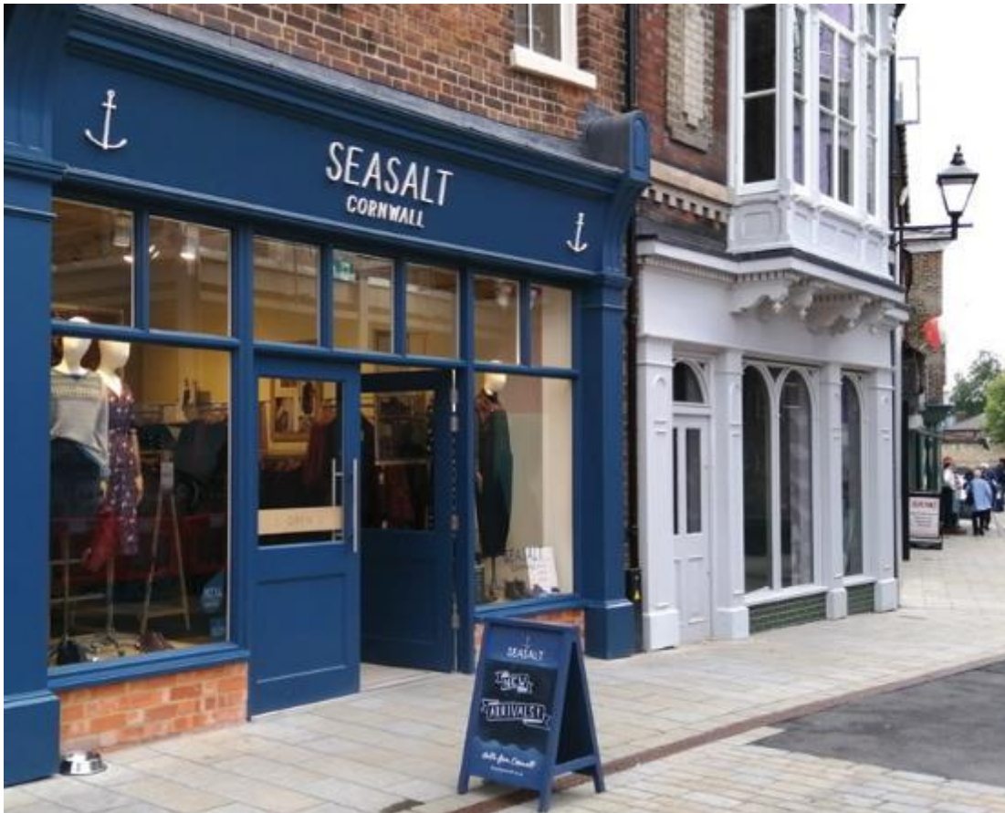
Figure 52 - The retention of original architectural features is key to safeguarding local character
