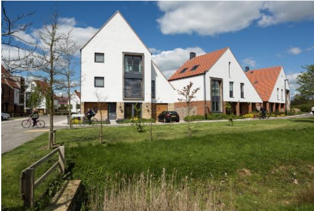
Figure 90 - Derwenthorpe Phase 1, Osbaldwick, York: An exemplar low-carbon community of energy efficient homes. A community heating system supplied by biomass boilers was chosen as the most cost effective and future-proof means of achieving low carbon emissions. Green infrastructure lies at the heart of the masterplan, with the open space shaped by flood prevention and landscaping for biodiversity.
