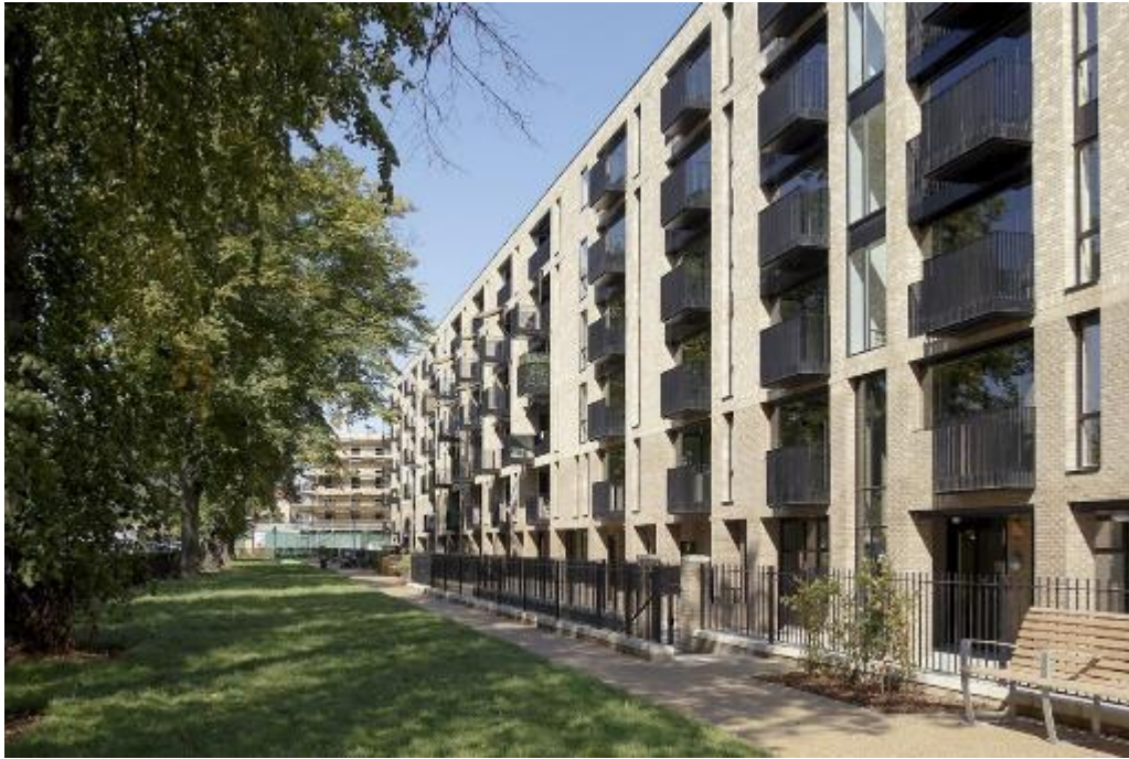
Figure 82 - Buccleuch House, Clapton: A mixed-tenure development providing homes for three different communities; first time buyers, Orthodox Jewish families and older people who need extra care. The design creates one unified building with very little difference externally across the three tenures except for subtly different balcony types designed with the practical and cultural requirements of the residents in mind.
