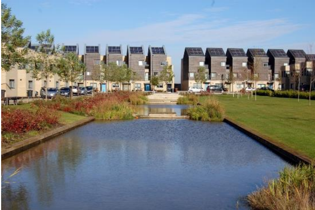
Figure 94 - Barking Riverside, East London: A 179 hectare brownfield site situated on the north bank of the River Thames with planning permission granted for over 10,000 homes. Over 40% of land is dedicated to open space including parkland linked by cycle routes and footpaths. A range of environmental measures include energy saving homes, rainwater harvesting, SUDs, green roofs, and conservation of local biodiversity.
