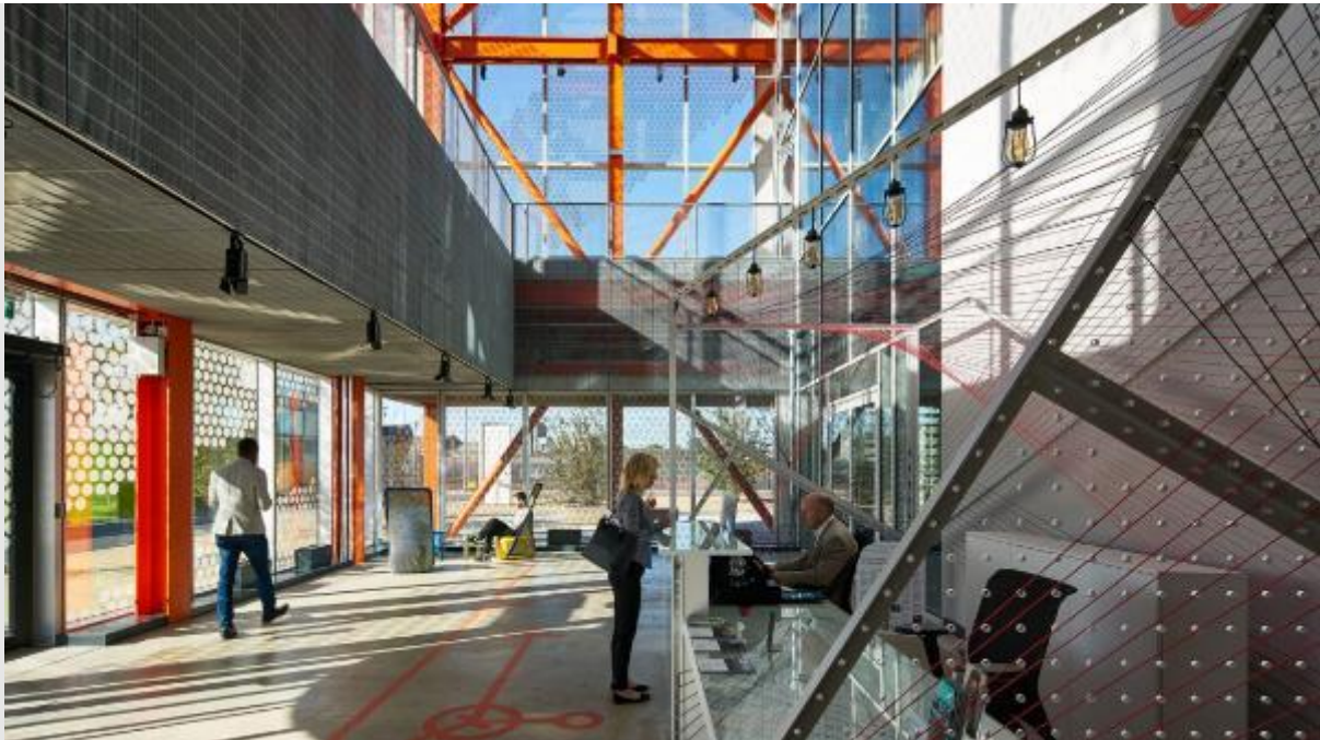
Figure 49 - Here East, Stratford: The refit of the London 2012 Media Centre into commercial space for creative and digital industries was inspired by the light industrial factories and yards of neighbouring Hackney Wick. The aim was to make a series of huge buildings more social, dynamic and flexible with the potential to evolve. The original windowless facade was removed to create a glazed outer layer of flexible work, studio and commercial spaces around the perimeter - maximising natural daylight, ventilation and views. Education, employment and enterprise coexist behind colourful animated facades featuring projecting/inset balconies with bright orange metalwork, brise soleil, and solar dot patterned glazing. The combination of elements is effective in breaking down the scale of the building.
