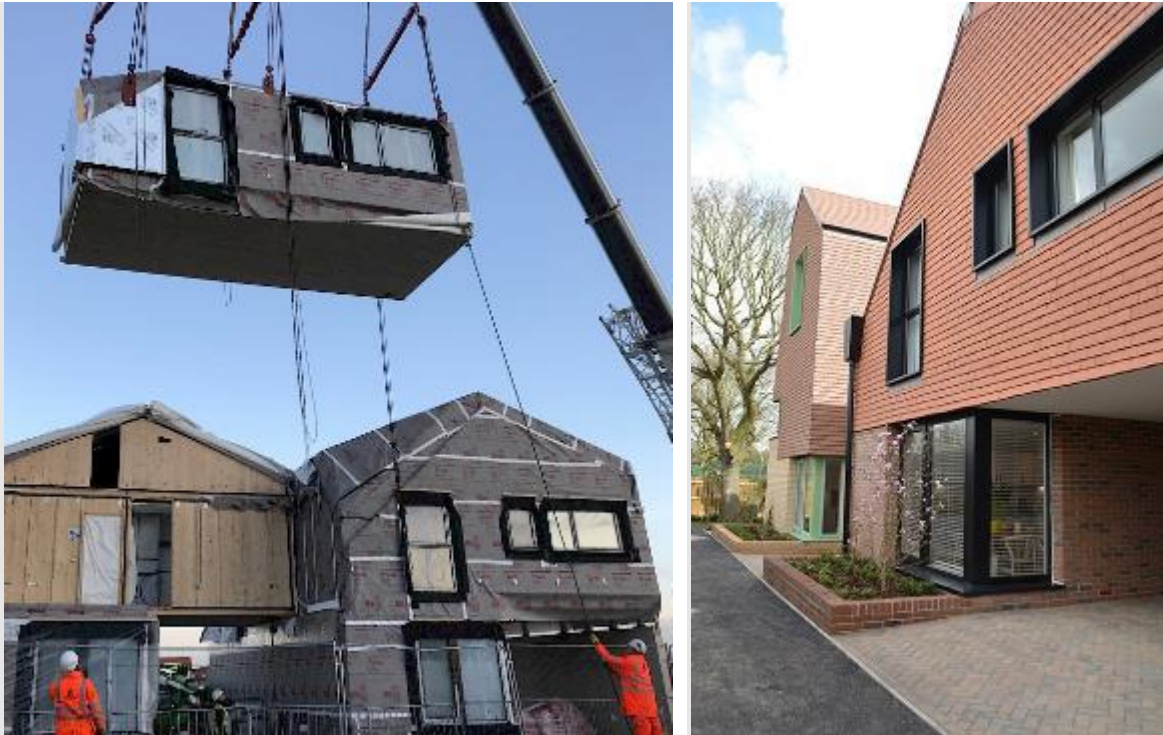
Figure 92 - Beechwood West, Basildon: A new neighbourhood of over 250 volumetric family houses utilising factory-built modular technology offering a choice of housing typologies, layouts and external finishes, precision engineered in an efficient and sustainable way with a significant reduction in construction waste compared with traditional build methods.
