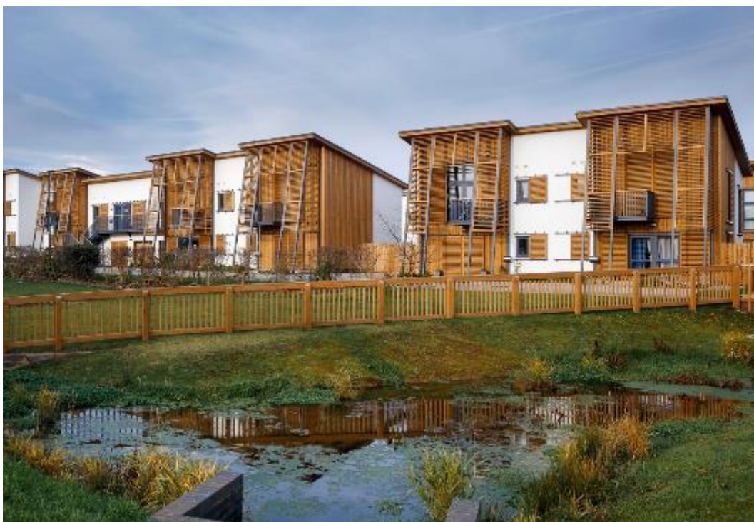
Figure 91 - Hanham Hall, South Gloucestershire: 187 homes built from factory made elements which minimise waste and are energy efficient to produce and build, the zero-carbon standard is achieved by using an efficient building envelope constructed using Structural Insulated Panels (SIPs) and roof-mounted PVs. The homes combine stack and cross ventilation, large openings, deep roof overhangs, balconies and shutters to avoid overheating.
