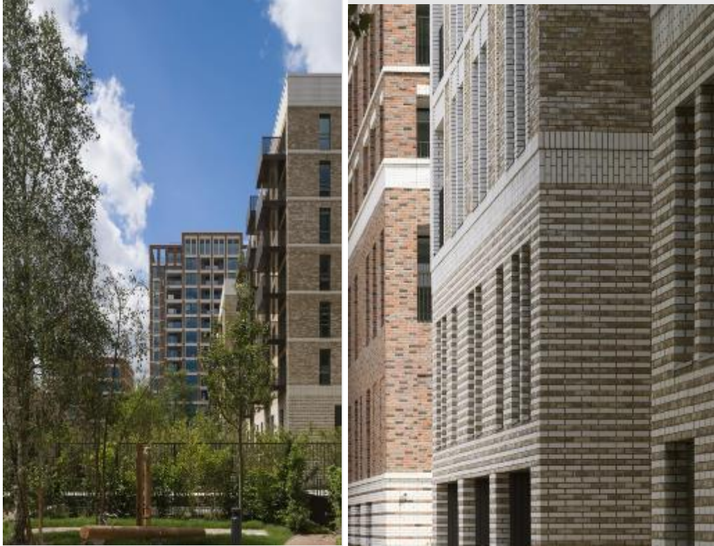
Figure 18 - Elephant Park, London: Creates a distinctive neighbourhood comprising of townhouses, mansion blocks and a 16-storey tower; executed in blends of five different bricks creating a playful, decorative effect which breaks down the volume of the large-scale blocks.
